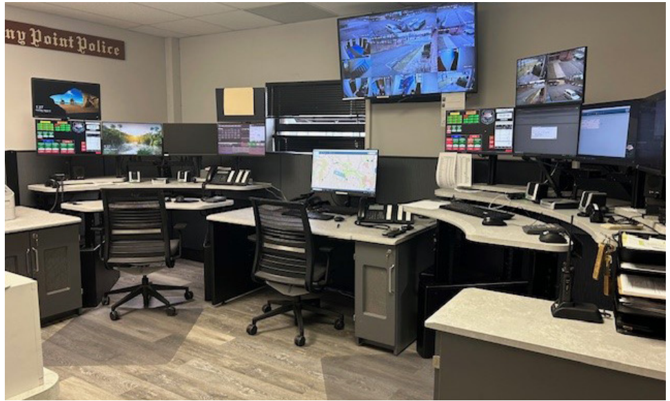
The newly renovated Dispatch Center located at the Stony Point Police Department.
